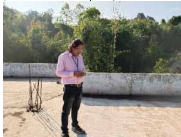
Mawpdang Village [Ch; 11+680] (On the roof of Minot Secondary School)
