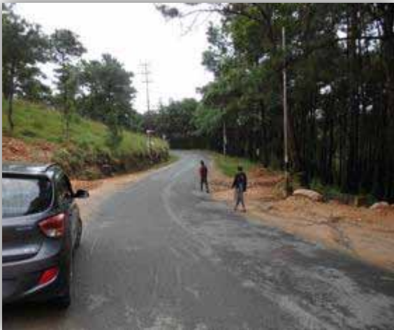
Photo: Road section near start point (at km 2+510)
