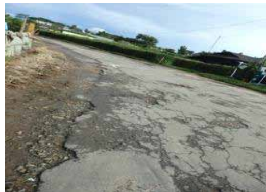
Photo: Road conditions at km 7+810
