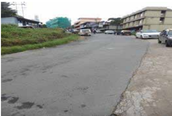
Photo: Road conditions at km 4+400
